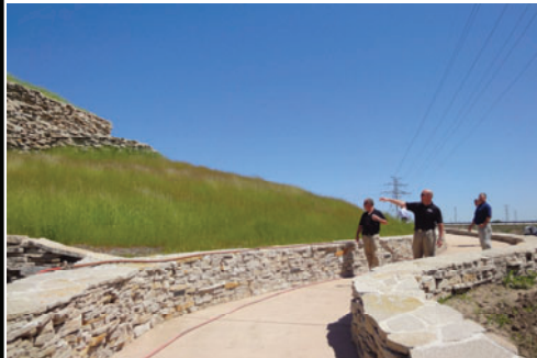
The sloped walkway leads to the observation deck and appears to be part of the natural hillside.
