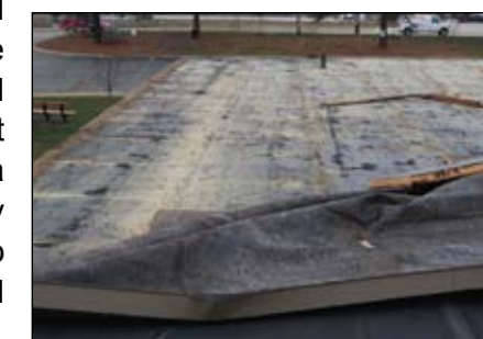
Wind damaged EPDM roof system over Center for Creative Learning - Ellisville, MO
