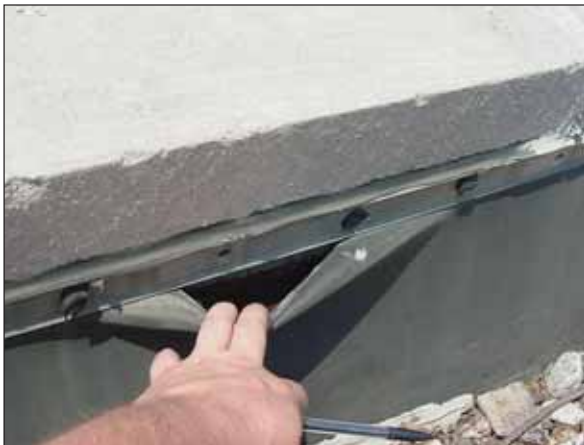
Detecting source of water infiltration in parapet wall during roof inspection
